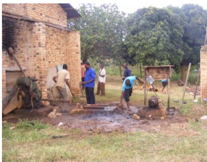
Pulling 190 ft deep water pipe
