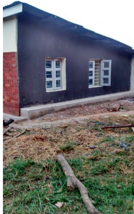
Milk barn - New windows and outer walls
