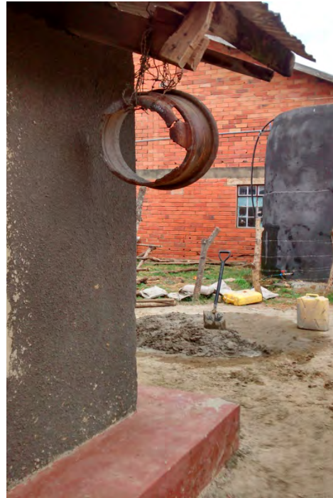
Milk barn - Upgraded exterior wall
