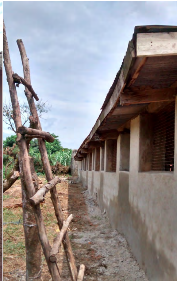
Milk barn with outside wall restored and foundation reinforced - note deteriorated roof
