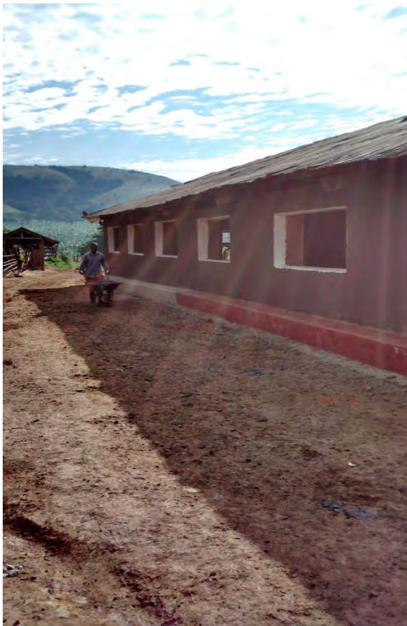
Milk barn with outside wall restored and foundation reinforced - note deteriorated roof
