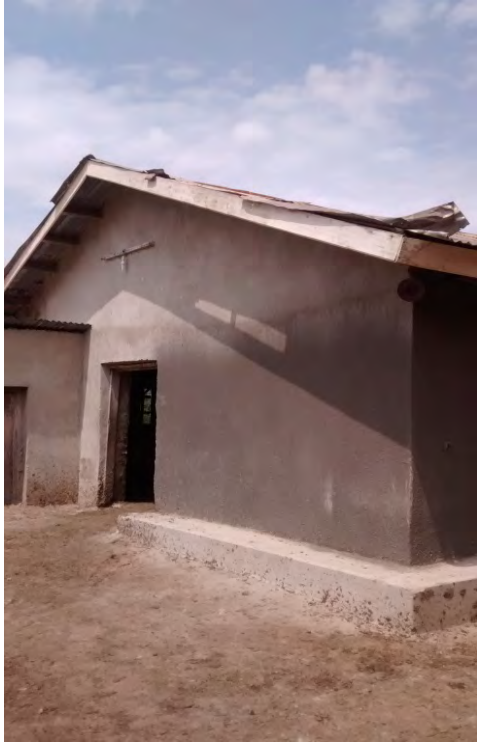
Milk barn -Exterior walls upgraded - 6/2014
